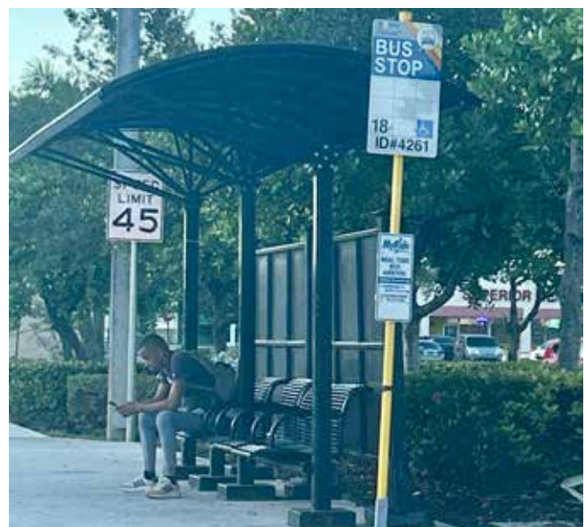
Image 27. Bus Shelter on SR 7/US 441
