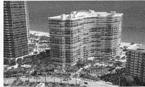
System Retrofit Majestic Towers Condo Bal harbor
