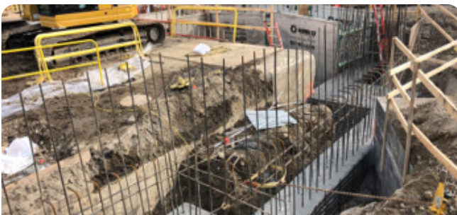
Clearview Pump Station Reconstruction, New York City DEP.
