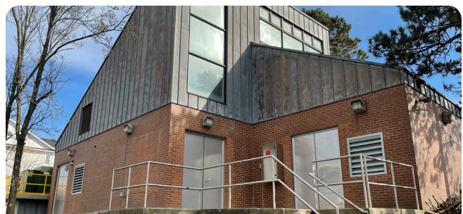
Roslyn Village, Morgan Park, and Shore Road Pump Stations, Flood Mitigation, Nassau County DPW.
