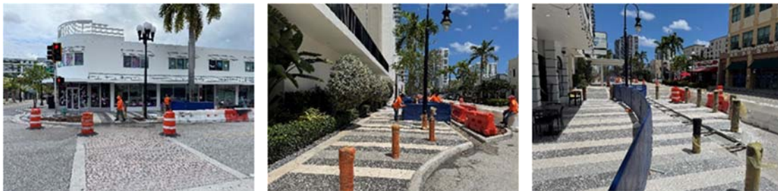
Phase IV – Pressure washing and sealing of pavers
