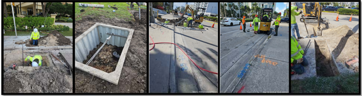
Horizontal Directional Drilling at A1A for electrical infrastructure and undergrounding work
