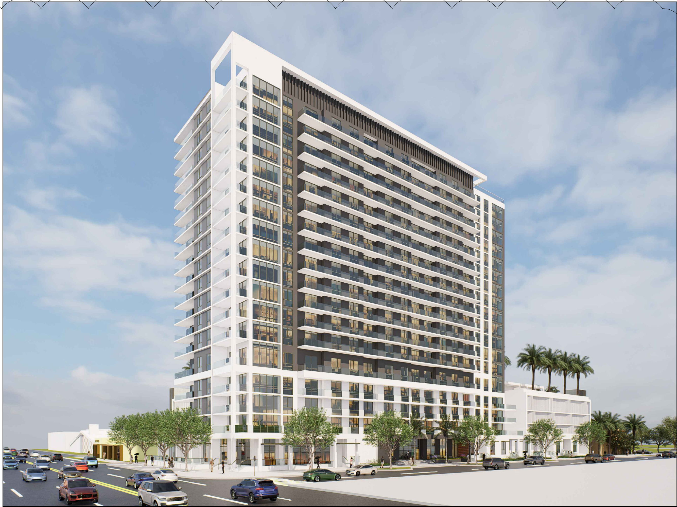
VIEW LOOKING NORTHEAST FROM FEDERAL HWY
