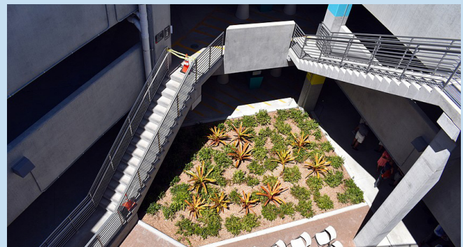
Image 35. St Armands parking garage.(Source: youobserver.com)
