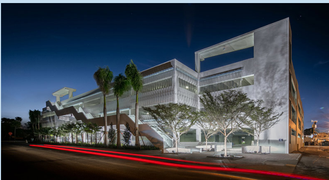
Image 34. St Armands parking garage.(Source: City of Sarasota)
