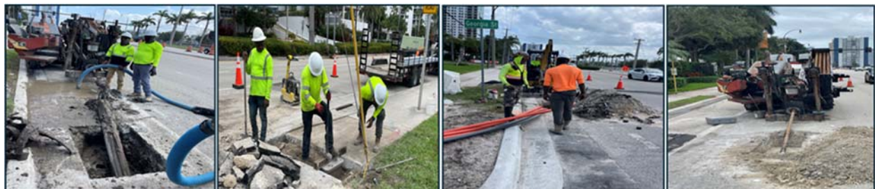
Horizontal Directional Drilling at A1A for electrical infrastructure and undergrounding work
