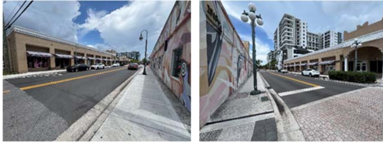
S. 20 th Avenue Improvements – pavement markings and signage
