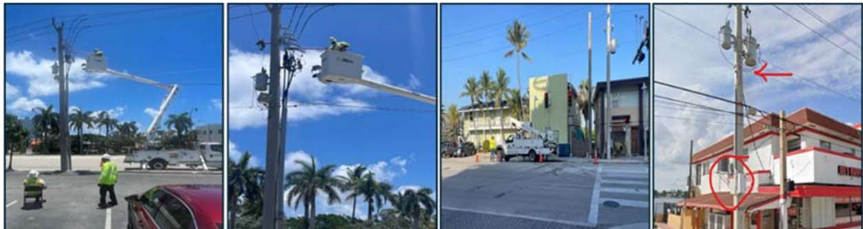
FPL system conversion from old system to new undergrounding infrastructure
