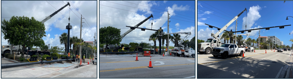
Mast arm installation
