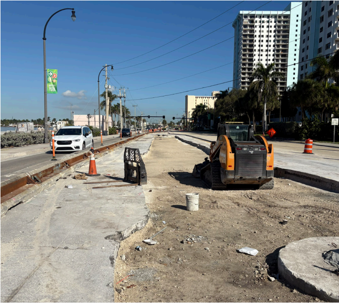
Early field investigations and constructability considerations inform design development (Azalea Project).
