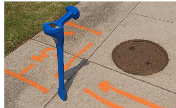
3D Utility Mapping Approach to eliminate utility conflicts during construction.
