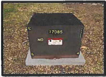
Typical Residential Pad-Mount Transformer Typical Size: 40"L x 36"W x 30"-41" H
