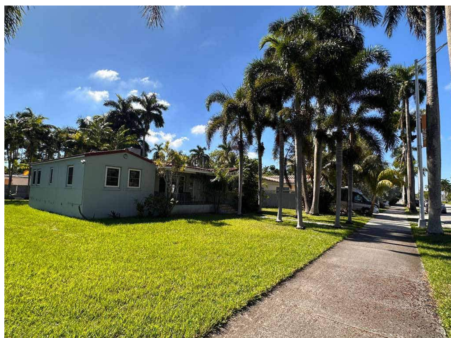
NORTHEAST CORNER VIEW
