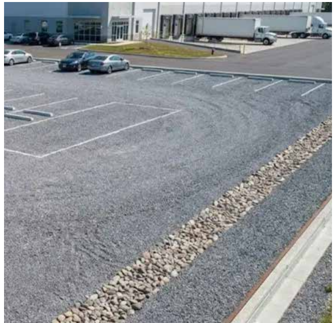
Image 31. Temporary gravel lot example.(Source: basecore)
