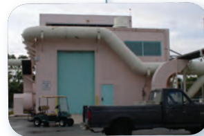
City of Hollywood Regional WWTP Influent Pump Station Upgrade $8.12 million
