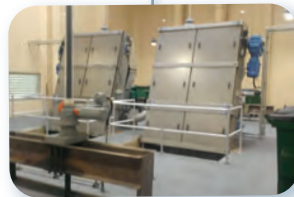
City of Hollywood SRWWTP Headworks Rehabilitation and Replacement $6.24 million
