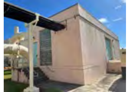
Existing IPS Control Building
