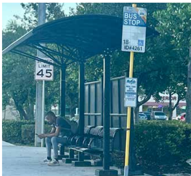
Image 27. Bus Shelter on SR 7/US 441
