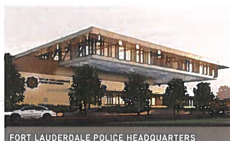
FORT LAUDERDALE POLICE HEADQUARTERS
