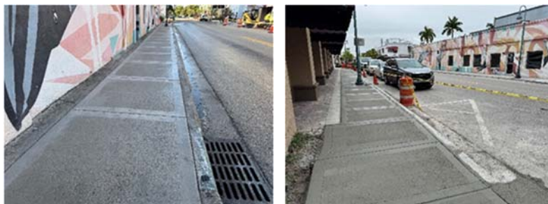
S. 20 th Avenue – placement of picture-frame concrete sidewalks
