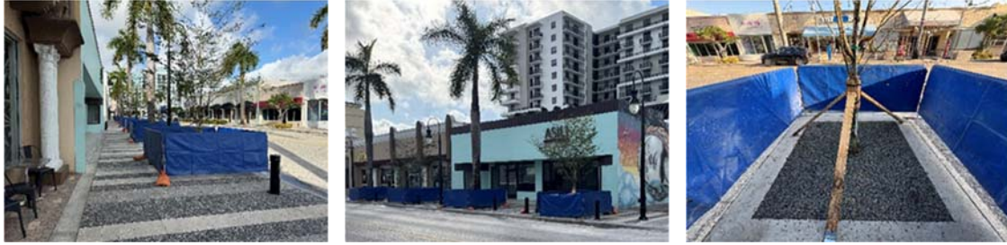
Phase III – installation of shade trees and Flexi-Pave
