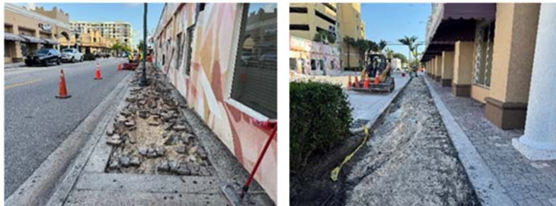
S. 20 th Avenue – demolition of sidewalks
