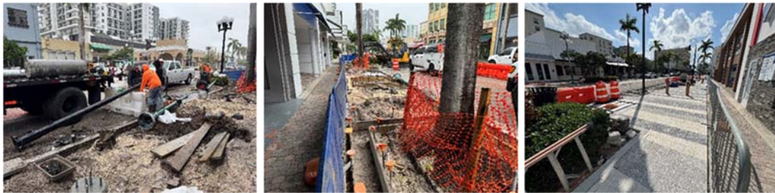
Phase IV – construction progress
