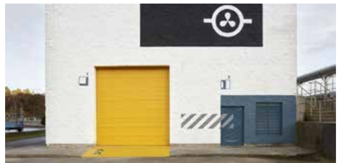
Image 05. Facade Improvement Program (PIP) Example. (Source: Pinterest)
