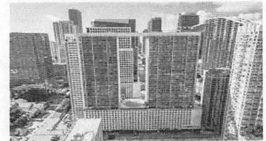
Repairs and Retrofits Brickell 500
