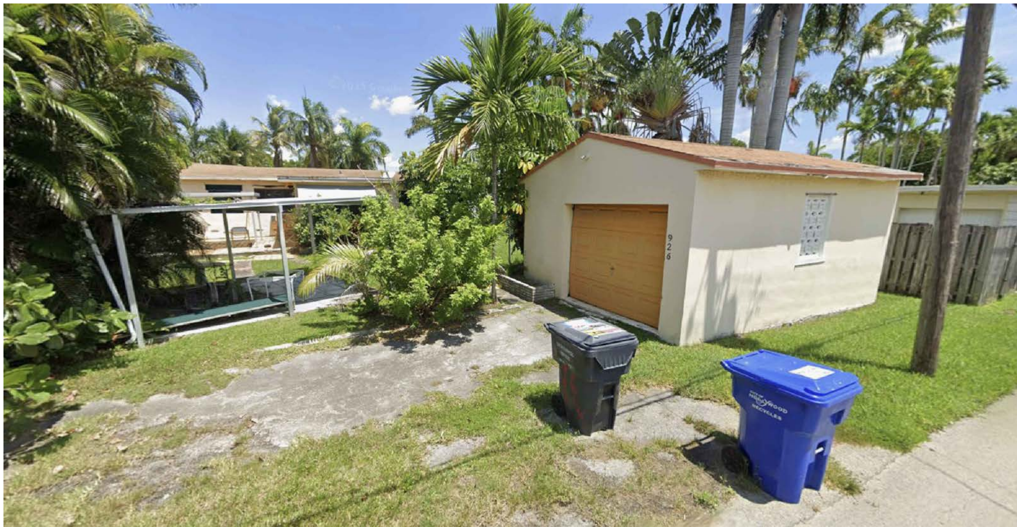
Rear of Home (Alley)
