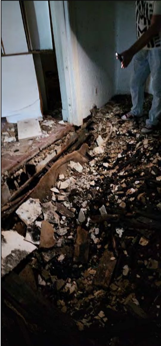
COLLAPSE OF FIRST FLOOR AND DETERIORATED MEMBERS
