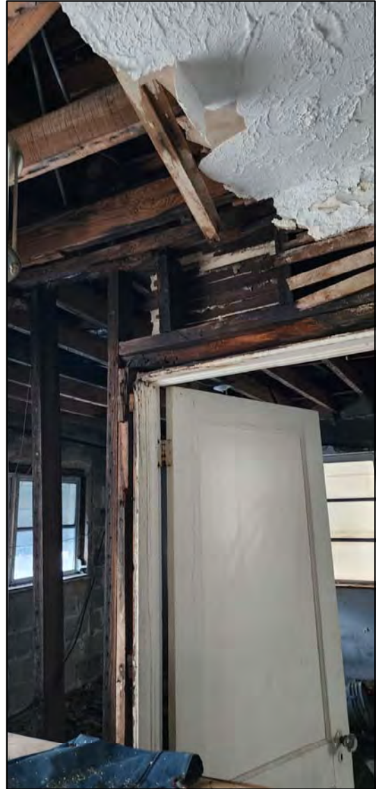
DAMAGED INTERIOR FRAMING
