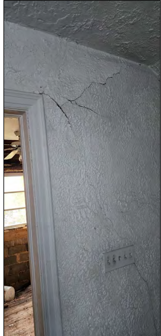
DIAGONAL CRACKS ABOVE THE DOOR
