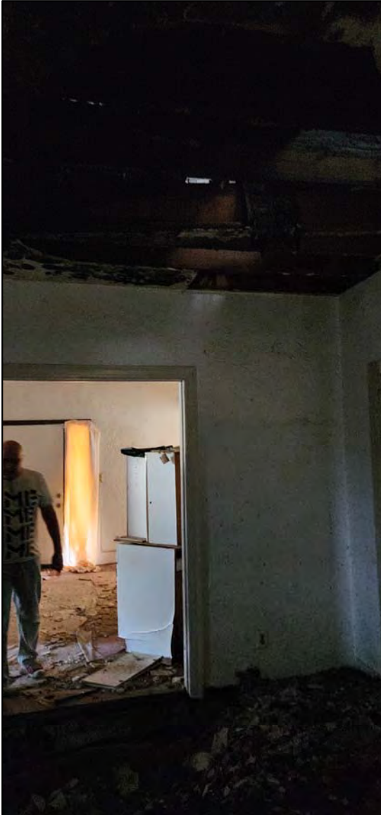
COMPLETE COLLAPSE OF FIRST FLOOR
