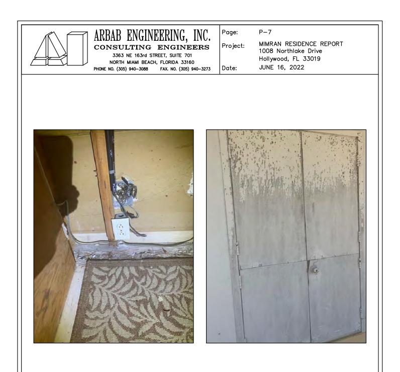
DETERIORATION OF WOOD FRAME AND IMPROPER ELECTRICAL WIRING. BADLY DETERIORATED EXTERIOR WOOD DOOR FACING SWIMMING POOL AND POOL DECK.
