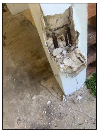
BADLY DAMAGED CONCRETE COLUMN WITH EXPOSED DETERIORATED REINFORCING
