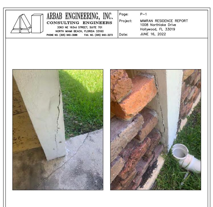
CONCRETE COLUMN AND FLOOR CRACK CONCRETE COLUMN CRACK ADJACENT ADJACENT TO THE GARAGE
