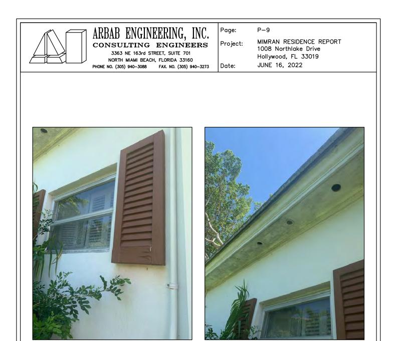
IMPROPER ATTACHMENT OF WINDOW AND GAP UNDERSIDE OF WINDOW FRAME DETERIORATED SOFFIT WITH POOR VENTILATION
