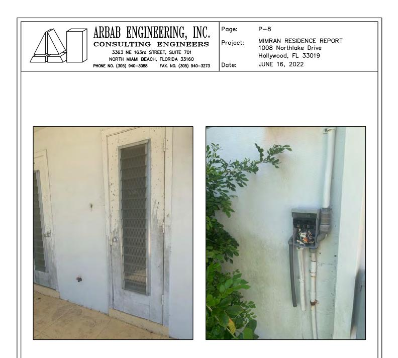
BADLY DETERIORATED WOOD DOOR FACING SWIMMING POOL
