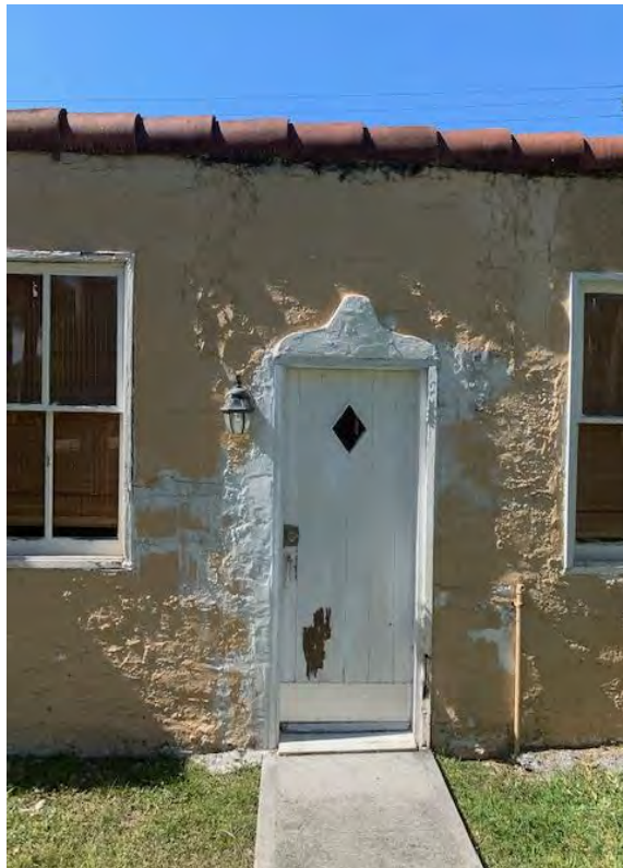
Deterioration of exterior wall
