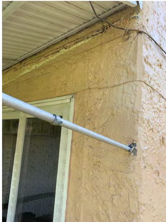
Wall crack
