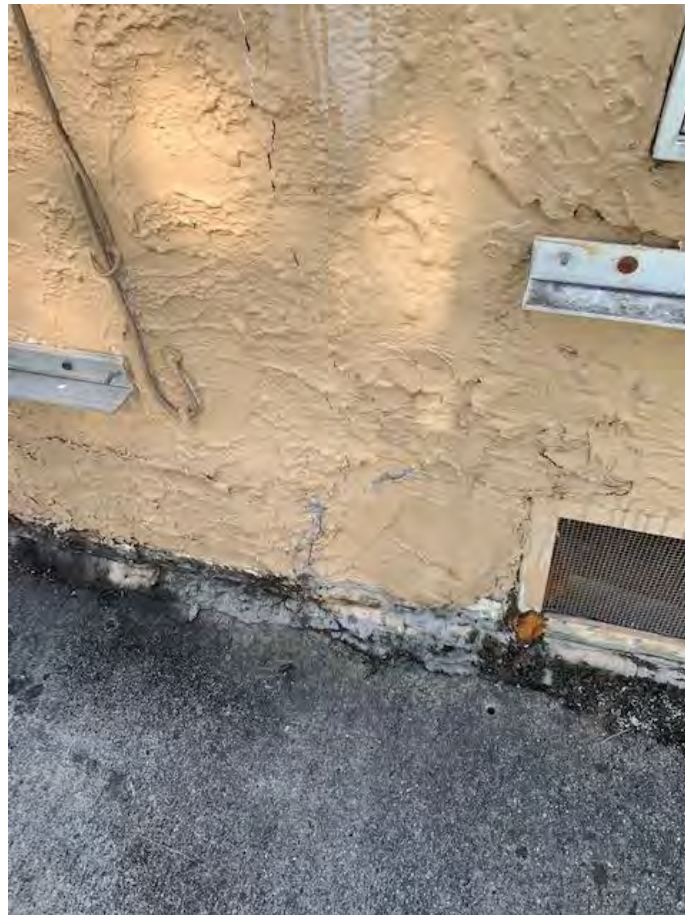
Erosion adjacent to footing
