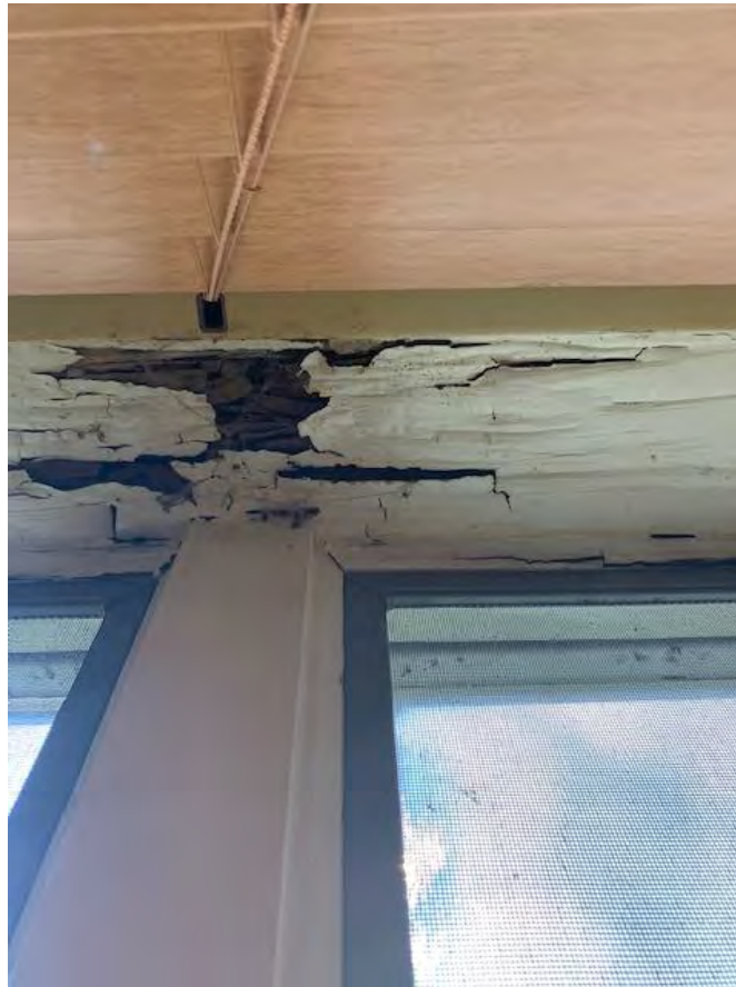
Deteriorated wood members
