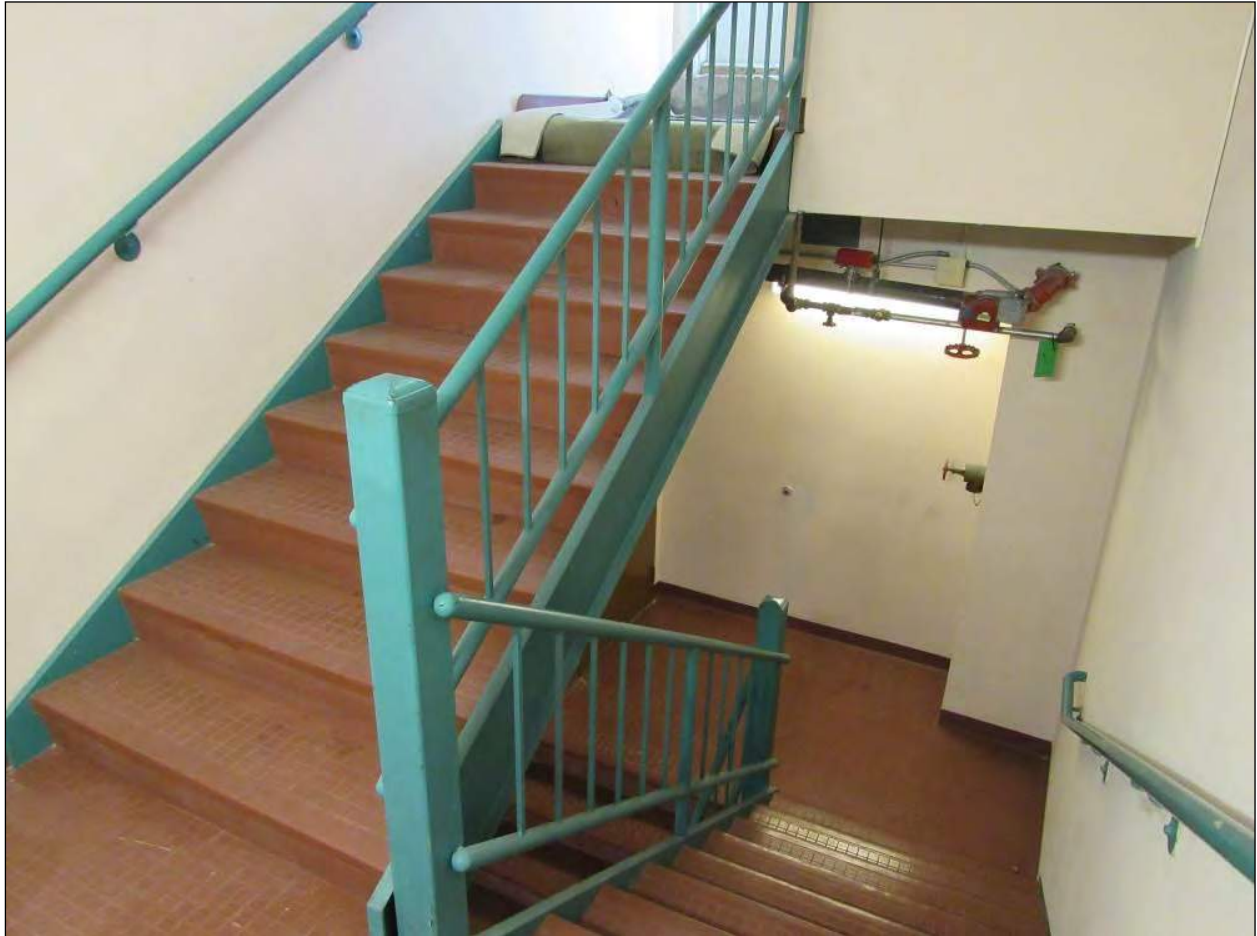
Figure 33. Interior staircase that was redone in the 1980s, with no historic fabric remaining, facing southwest.
