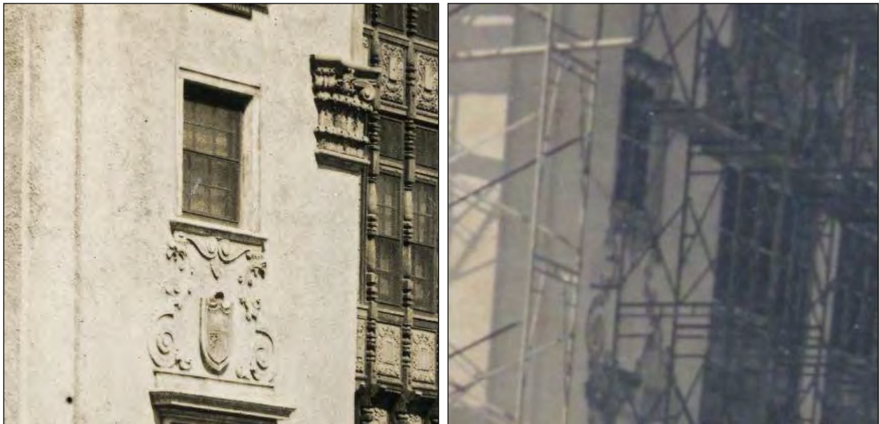
Figure 14. A comparison of the 1920s photograph (left) with the 1940s photograph (right) showing the decorative sill relief being removed from the façade.
