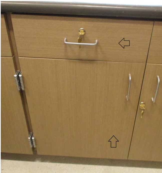
Image 1: Laminate installed improperly. The cabinet door's grain/pattern is oriented north and south and the drawer's grain/pattern is oriented east and west.
