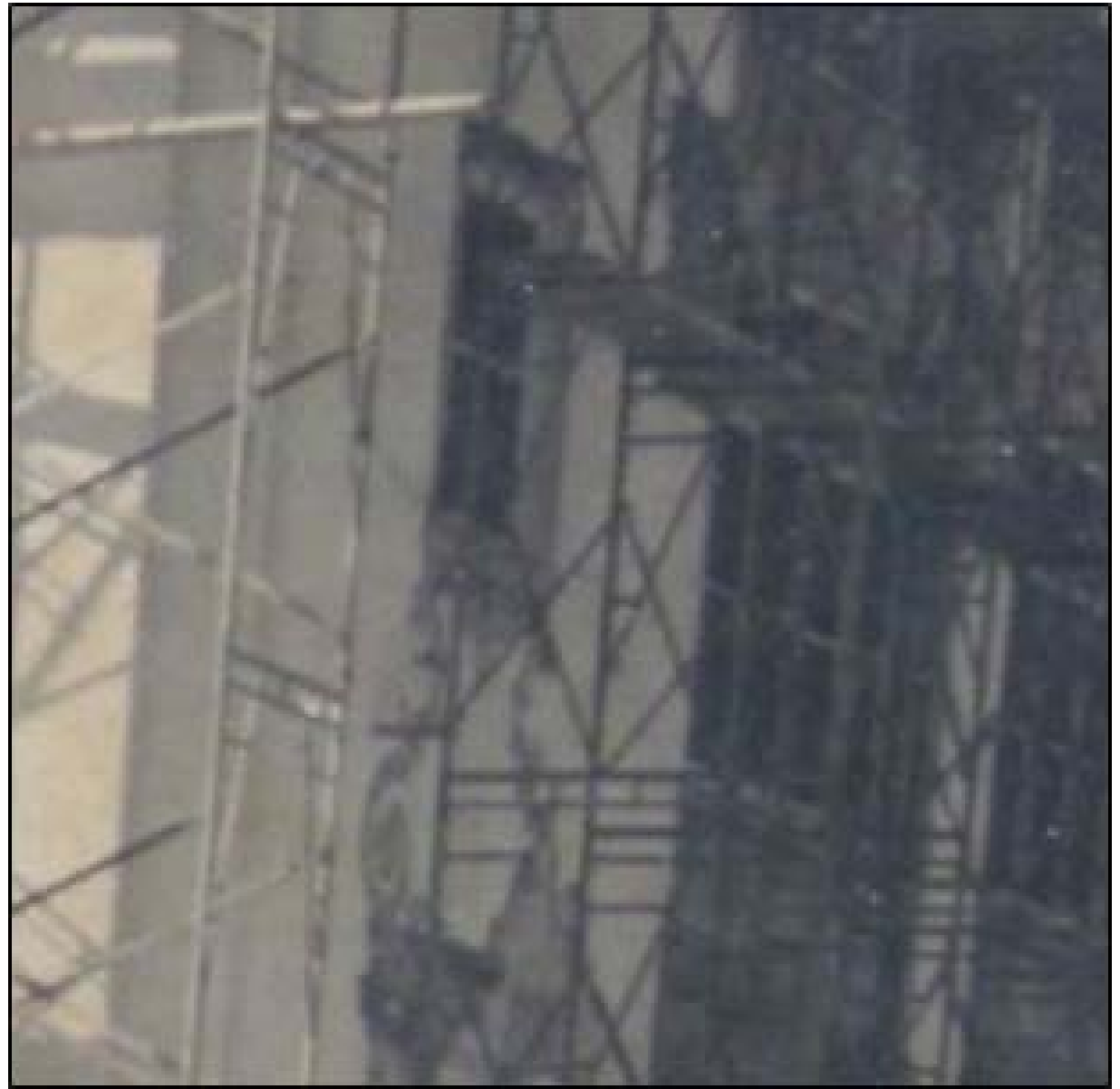
Figure 14. A comparison of the 1920s photograph (left) with the 1940s photograph (right) showing the decorative sill relief being removed from the façade.
