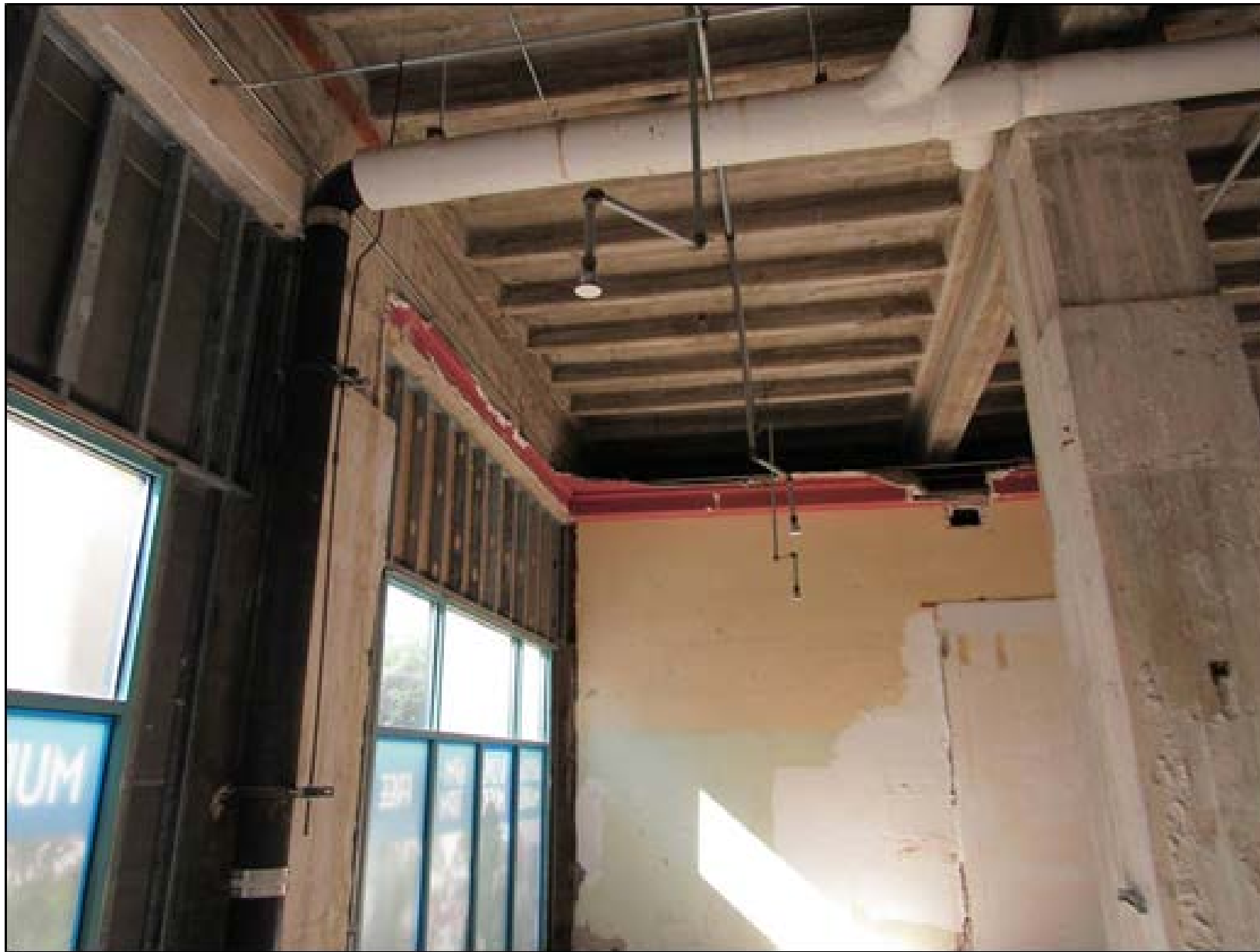
Figure 28. The southwest corner section of the original plaster molding, visible here in red, is all that remains of the original ceilings, facing west.
