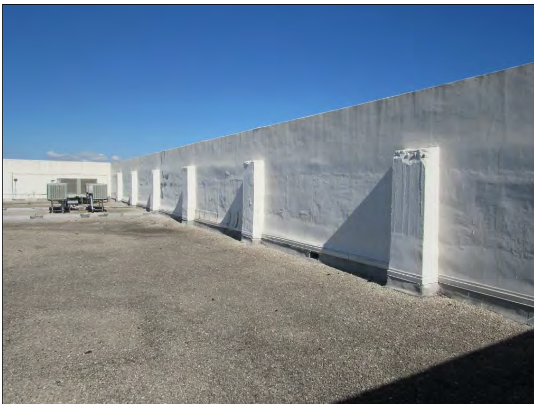
Figure 35. Cut pilaster extensions visible on the roof, facing northeast.
