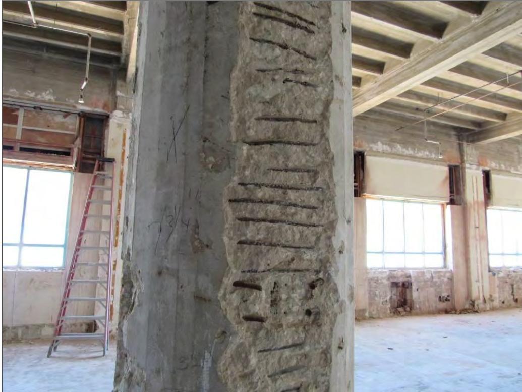
Figure 27. Close-up view of damage on one of the interior columns, with the metal rebar clearly visible, facing southeast.
