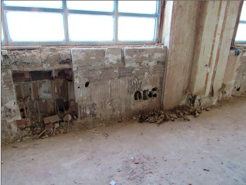
Figure 36. Poor condition of infill at the bottom of one of the eastside windows, facing southeast.
