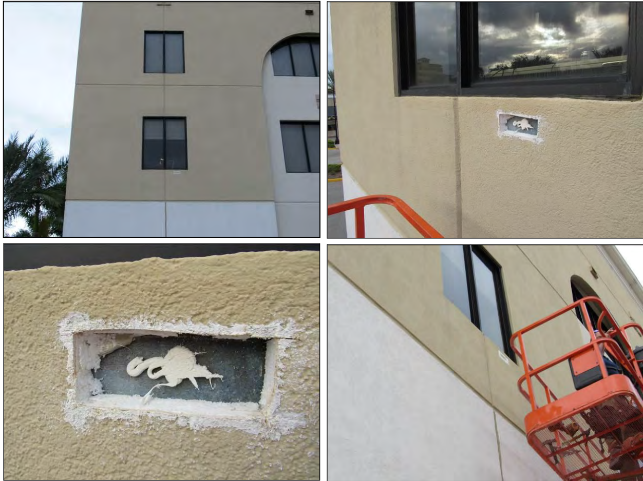
Figure 38. The removal of the EIFS and the smooth concrete visible underneath confirms the removal of the original decorative sill that was once located below this eastside window.
