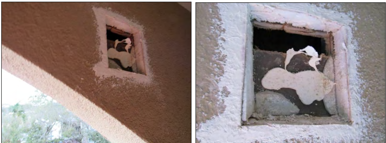
Figure 39. The removal of the EIFS on one of the arches on the south elevation reveals modern plywood and metal framing from the 1980s renovation used to imitate the original arches, which are no longer present.
