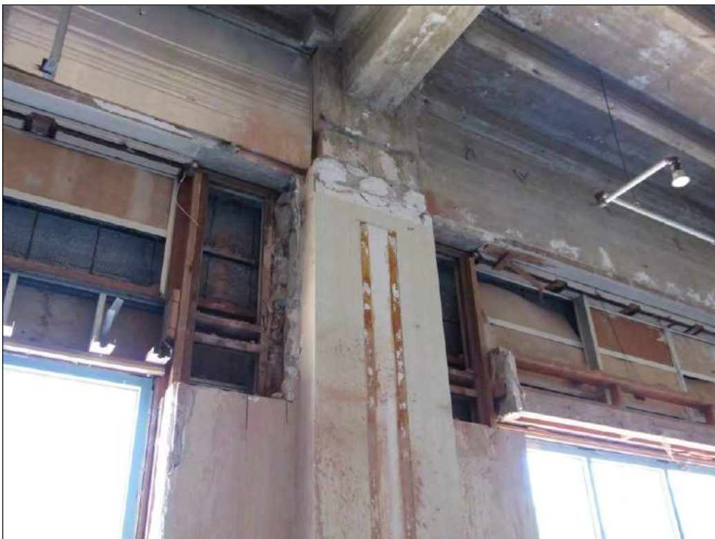
Figure 37. Tops of two of the windows located on the east side, with older wood and newer aluminum visible in the infilled section, facing southeast.
