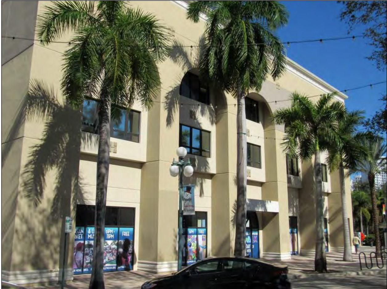
Figure 24. View of the five arched openings on the south elevation recreated in the 1980s, facing northeast.
