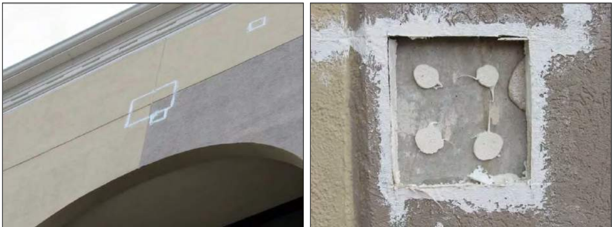
Figure 41. The removal of the EIFS and the smooth concrete visible in the former location of the decorative central medallion on the south façade also confirms the destruction of this once prominent feature.
