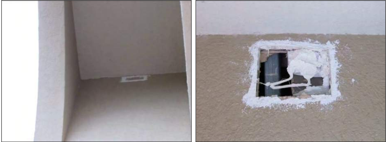
Figure 40. In this location where the arches meet the columns on the south elevation, the removal of the EIFS again shows modern plywood and metal framing with no historic fabric remaining.
