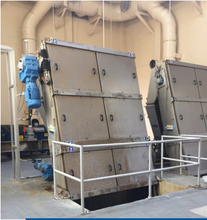
The influent screens at the SRWWTP are in good condition.
