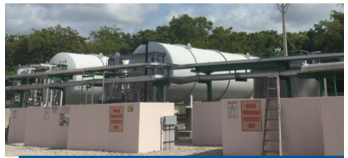
Existing high purity oxygen system (HPO) could be replaced with newer Vacuum Pressure Swing Adsorption (VPSA) technology with multiple advantages.
