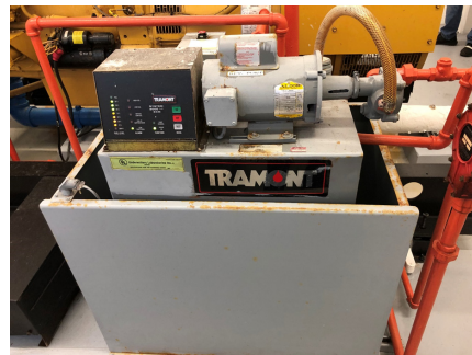
Existing Day Tank to be replaced.
