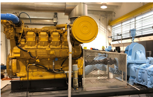
Emergency diesel driven pump that a new day tank will be provided for.
