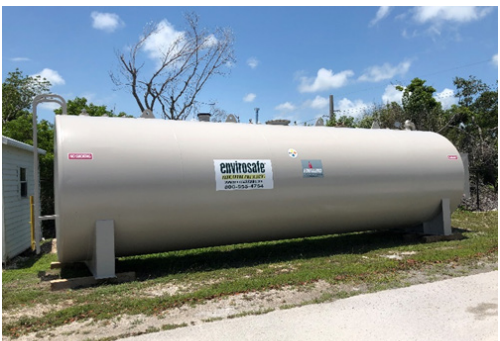
Owner supplied 10,000 gallon bulk fuel storage tank.
