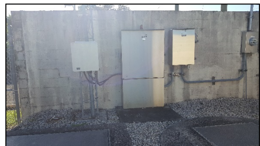
Existing Control Panel & RTU
