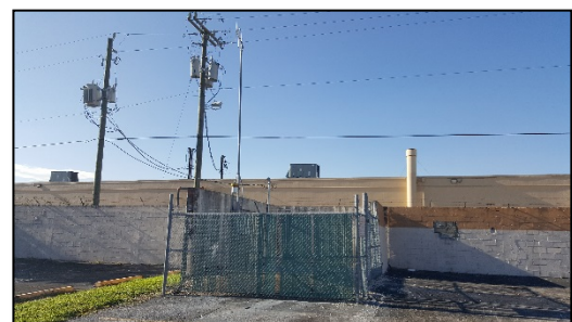
Existing FPL Pole Mounted Transformers
