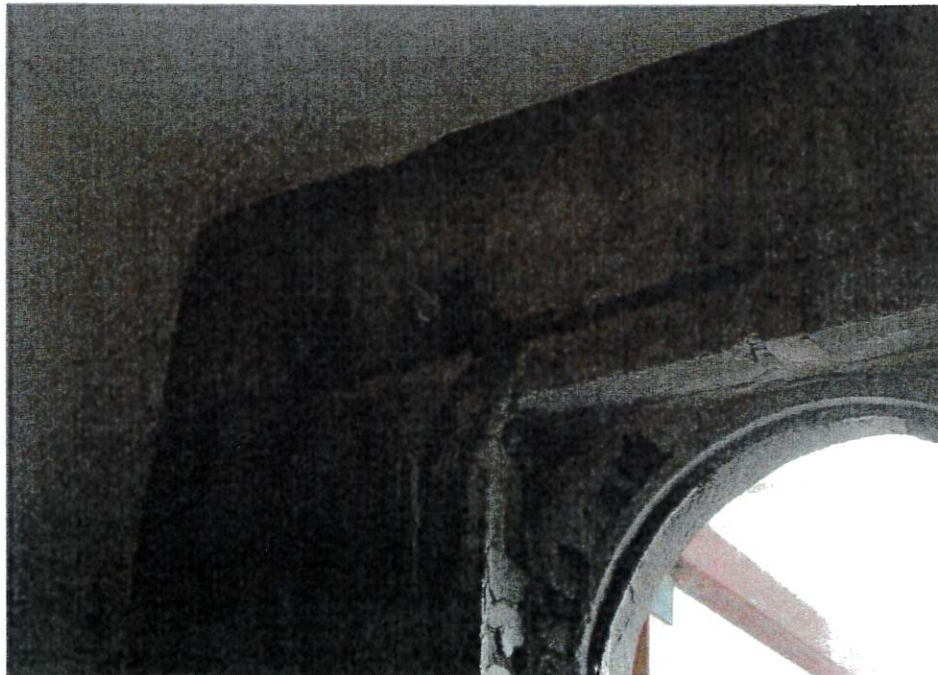
20. View of connecting rods for restoration placed in spalled concrete area with cracks and corroded reinforcement on the second floor of the structure.
