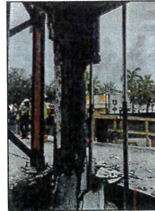
Column at south façade, other view. Observe Spalling and cracking at the base
