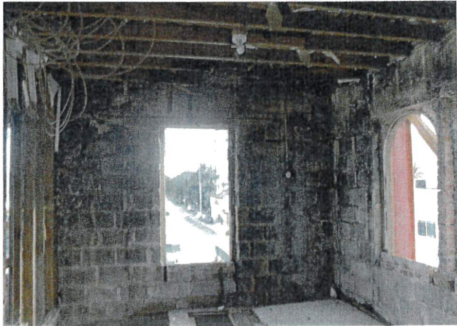
9. Interior view of the charred CMU walls, deteriorated wood floors and wood truss in the southwest corner of the structure, third floor level.
