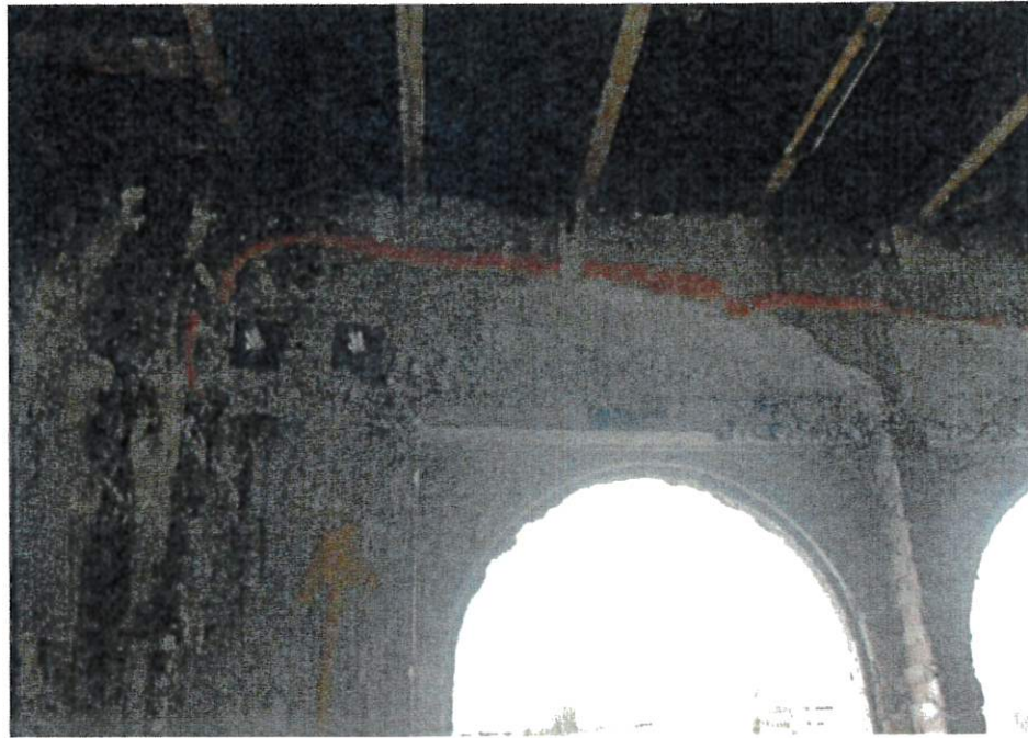
13. Typical view of the third level tie beam with cracked, spalled and honeycombed concrete and exposed corroded reinforcement at the north area of the structure.
