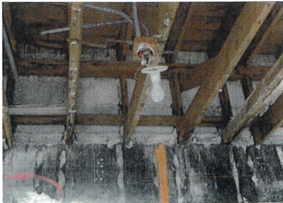
10. Interior view of deteriorated CMU parapet wall above tie beam in the southwest area of the structure, third floor level.
