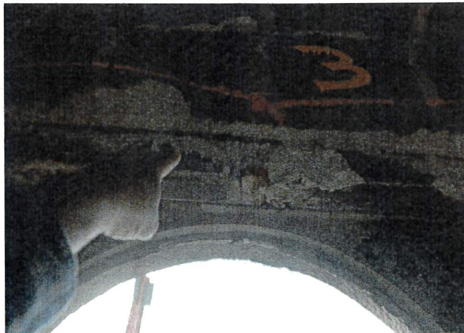
8. Typical view of the third level tie beam with cracked and spalled concrete and exposed corroded reinforcement at the southwest area of the structure.
