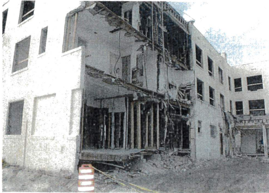
23. View of removed wall with exposed wood flooring, partition walls, stem wall and crawl space the ground floor level at the southeast area of the structure.
