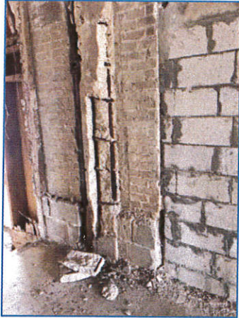
Column w/excessive spalling (W façade)
