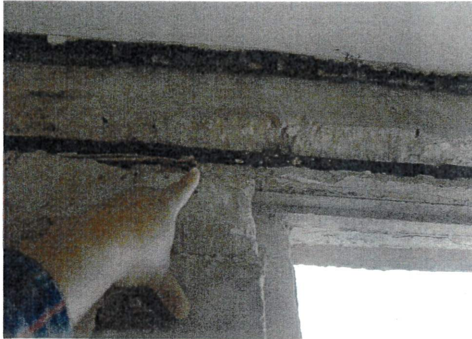
19. Close-up view of tie-beam with cracks and corroded reinforcement; west area of the second floor level.
