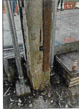
Column at south façade, with crack & spall at base
