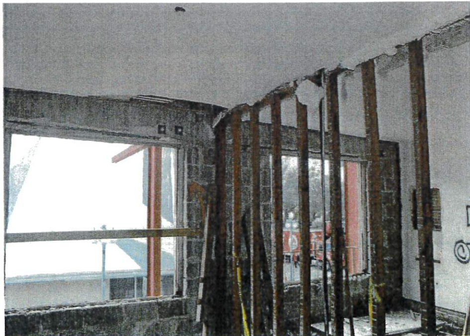
18. View of tie-beam with cracks and corroded reinforcement with connecting rods for the restoration; west area of the second floor level.
