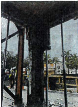
Top portion of same column – existing block infill supported by shoring
