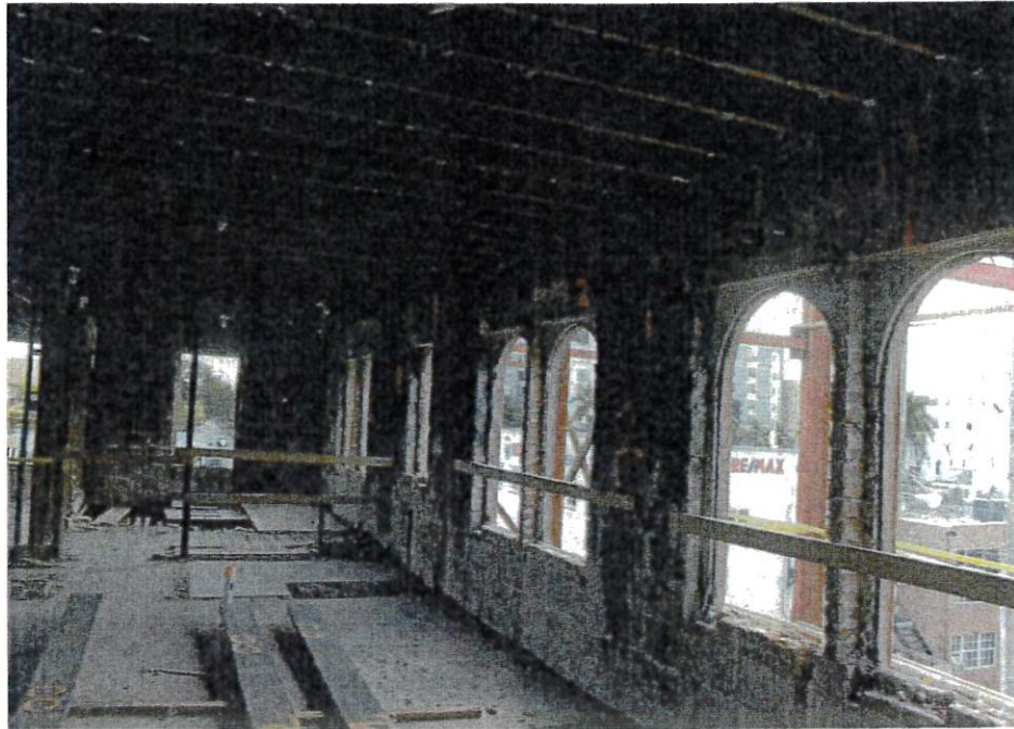
7. Interior view of the charred CMU walls, deteriorated wood floors and wood truss in the southwest area of the structure, third floor level.
