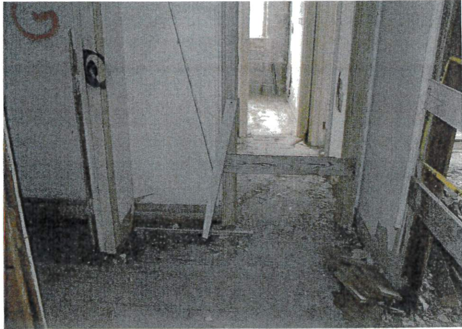
17. View of termite damaged deteriorated wood flooring with noticeable sloping and wall to floor separation in the corridor at the northwest area of the structure; second floor level.
