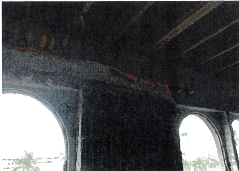
14. Typical view of the third level tie beam with cracked, spalled and honeycombed concrete and exposed corroded reinforcement at the north area of the structure.
