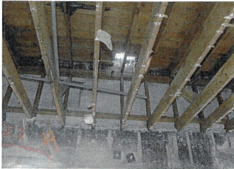
11. Interior view of deteriorated CMU parapet wall above tie beam in the west central area of the structure, third floor level; with rods in the tie beam and parapet wall above.
