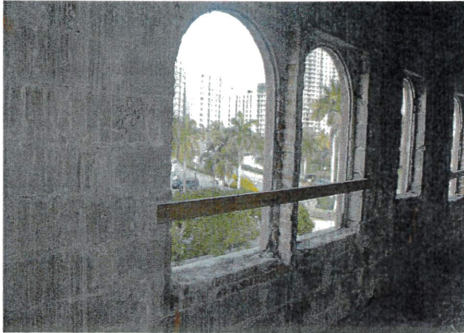
15. View of north wall with composite brick and CMU wall section on the third floor level of the structure,
