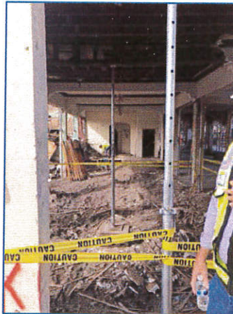
Sagged decorative beam (shored), wood joists to be shored (north portion)
