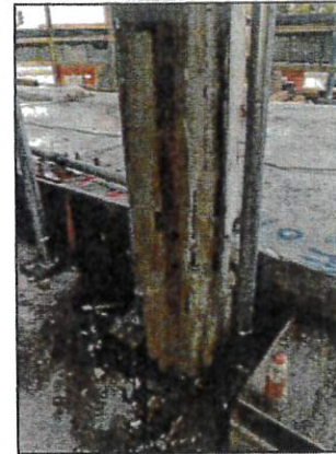
Column at south façade, other view. Observe Spalling and cracking at the base
