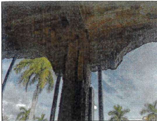
Top portion of same column – existing block infill supported by shoring
