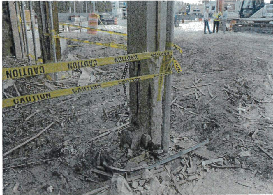
21. Typical view of column with cracked and spalled concrete sections and corroded reinforcement on the ground floor of the structure.
