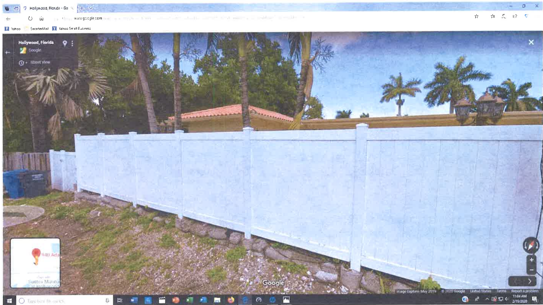
(3) 940 Adams Street-alley Built-up berm-no retaining wall for elevated fence 1 block west of 840 S Southlake Drive Renovation
