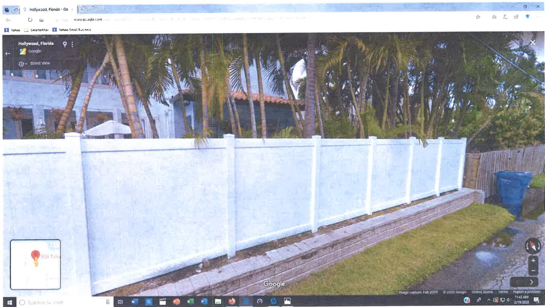
(6) 928 Tyler Street-alley New retaining wall not connected with elevated fence New Construction
