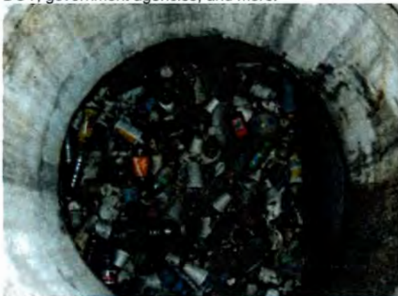
Before Sewer Cleaning
