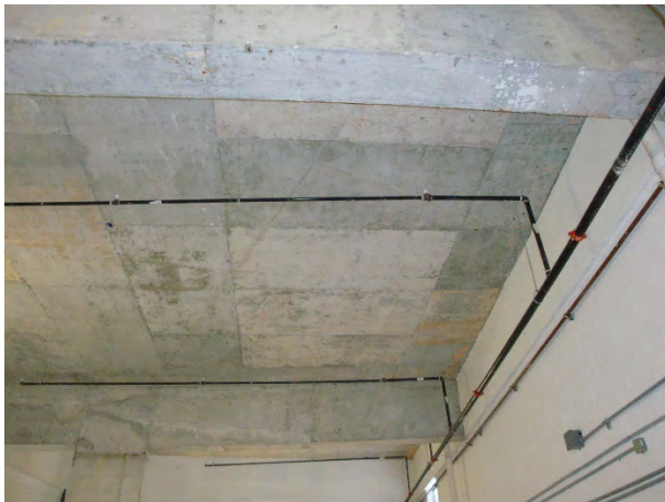
Fire Suppression System to be Relocated
