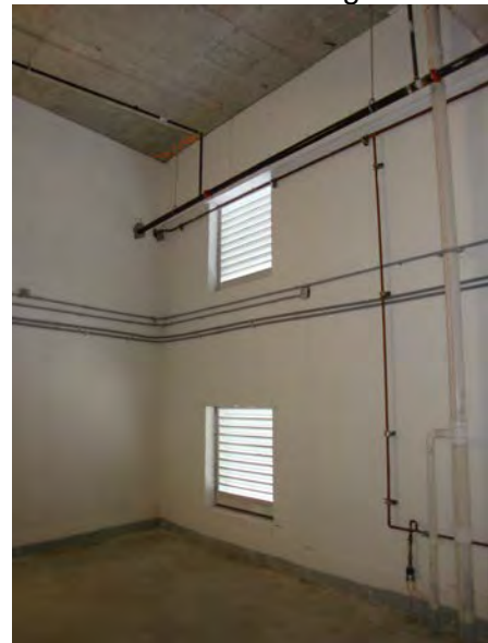
Vents near wall penetration location
