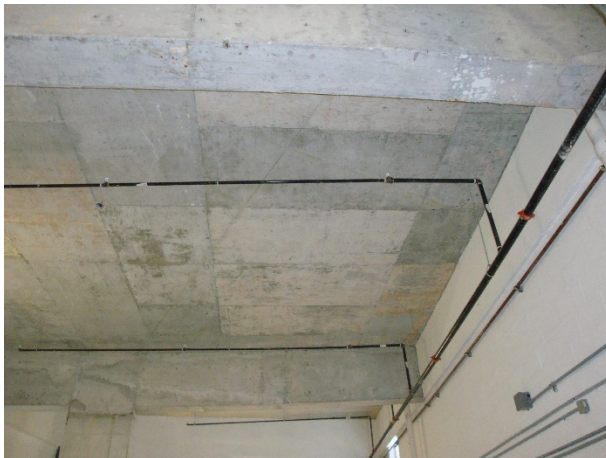
Fire Suppression System to be Relocated
