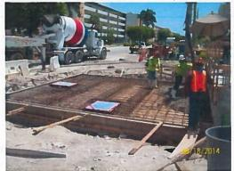
in the NE Quadrant of Hallandale Beach which required extensive public outreach to coordinate with the property owners. As a part of the design to collect the storm water 2 large storm water pump stations were installed in dewatered sheeted cofferdams that were 18 vertical feet below grade. The reinforced structures were cast in place because the size of the structures prohibited pre-casting. The
