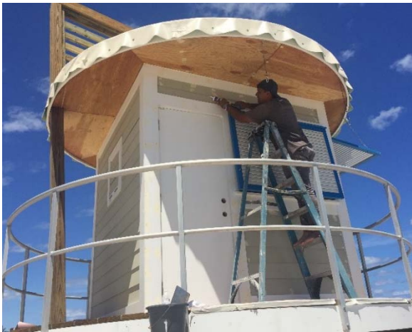
Application of caulking, First Aid Station
