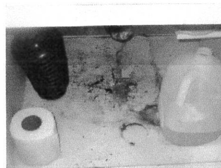
Photo #19 DAMAGED VANITY DUE TO DRAIN LEAK.
