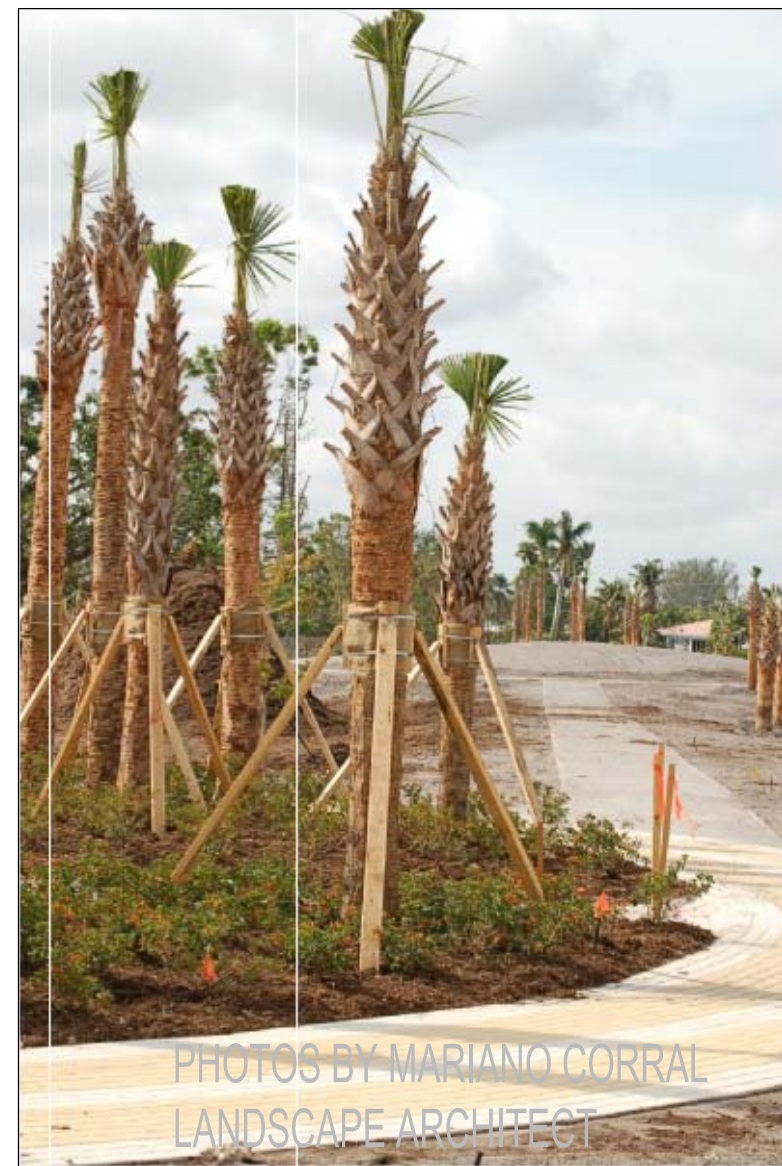
Use Four (4) wood planks 8' long to uphold palm tree over 22' height or 10' greywood and above.
