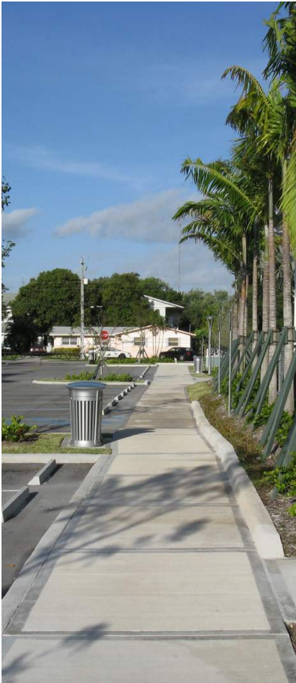
FIGURE 39 – PICTURE FRAME CONCRETE SIDEWALK
