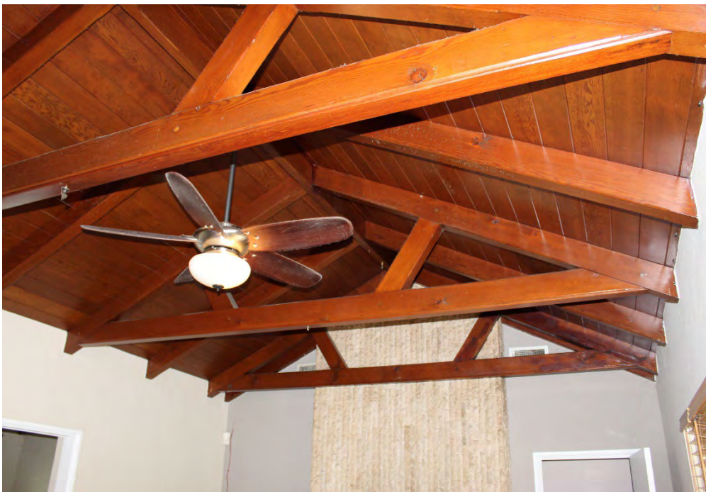
12. View of the sheathing, trusses and rafters over the living room of the residence.
