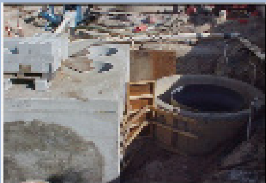
PCP diversion into Place and Existing Sewerage
