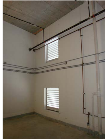
Vents near wall penetration location
