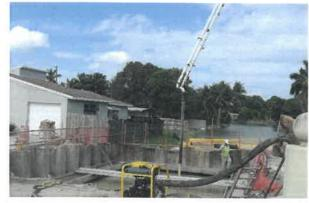
bottom for ground water control by tremie plug. Road Reconstruction included 0.4 miles of subbase, road base and 2" of asphalt. The rest of the neighborhood received 8,300 SY of Mill and over lay of 1". Pressure Pipe Stormwater Force Main included 3,472 LF of DIP ranging in size from 24 to 60 inch.
