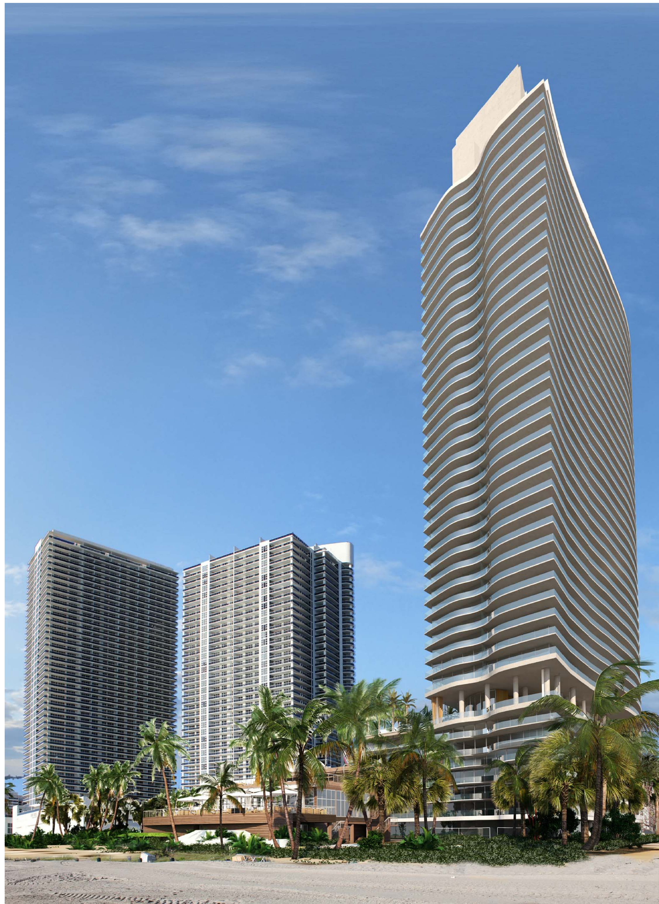
VIEW LOOKING SOUTHWEST
