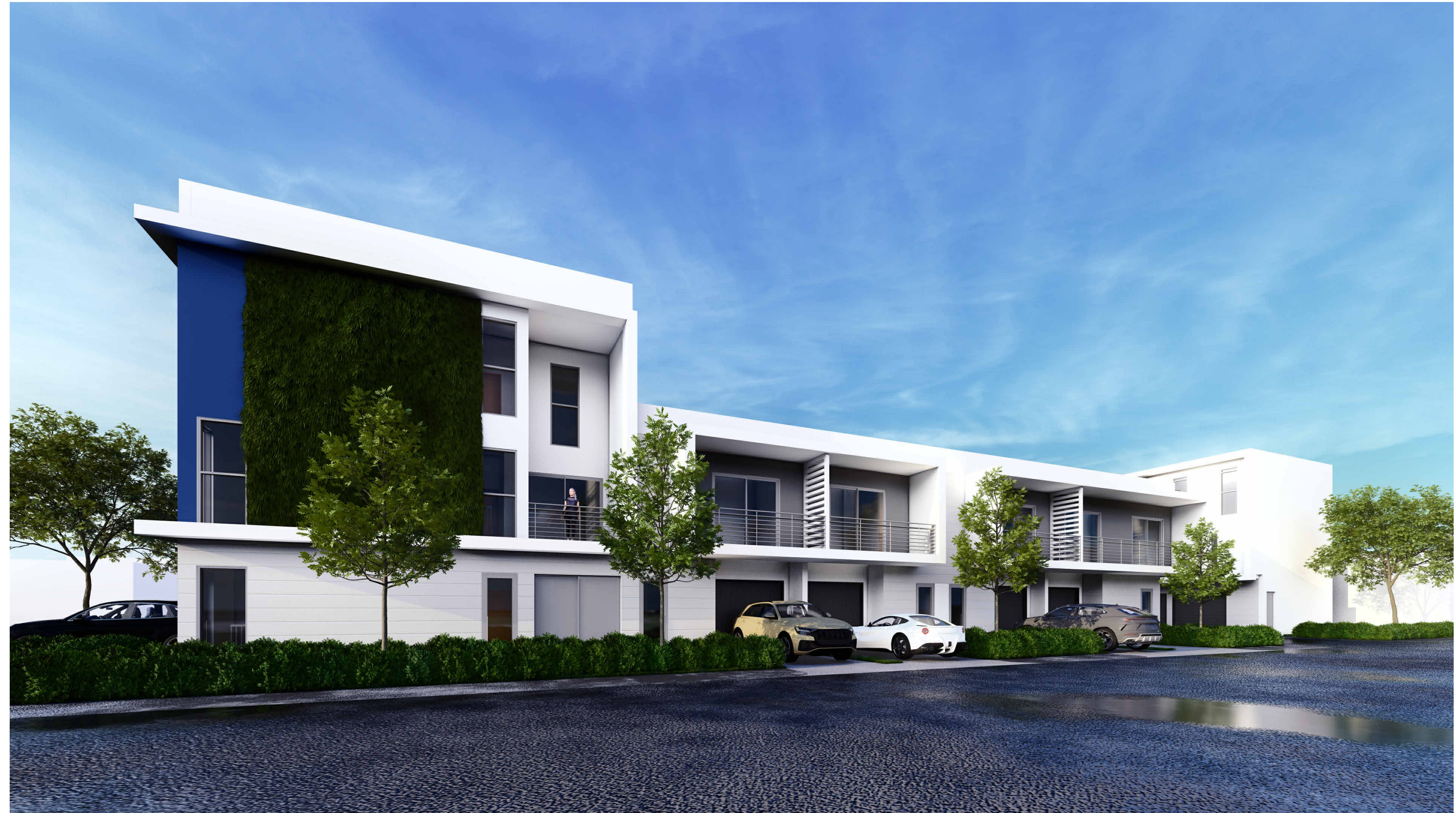
VIEWING NORTH (FROM LINCOLN STREET)
