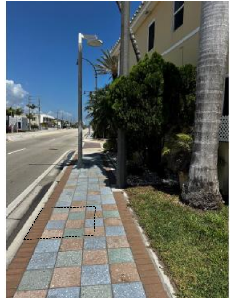
3. Cover tree grate with pavers until a solution is identified
