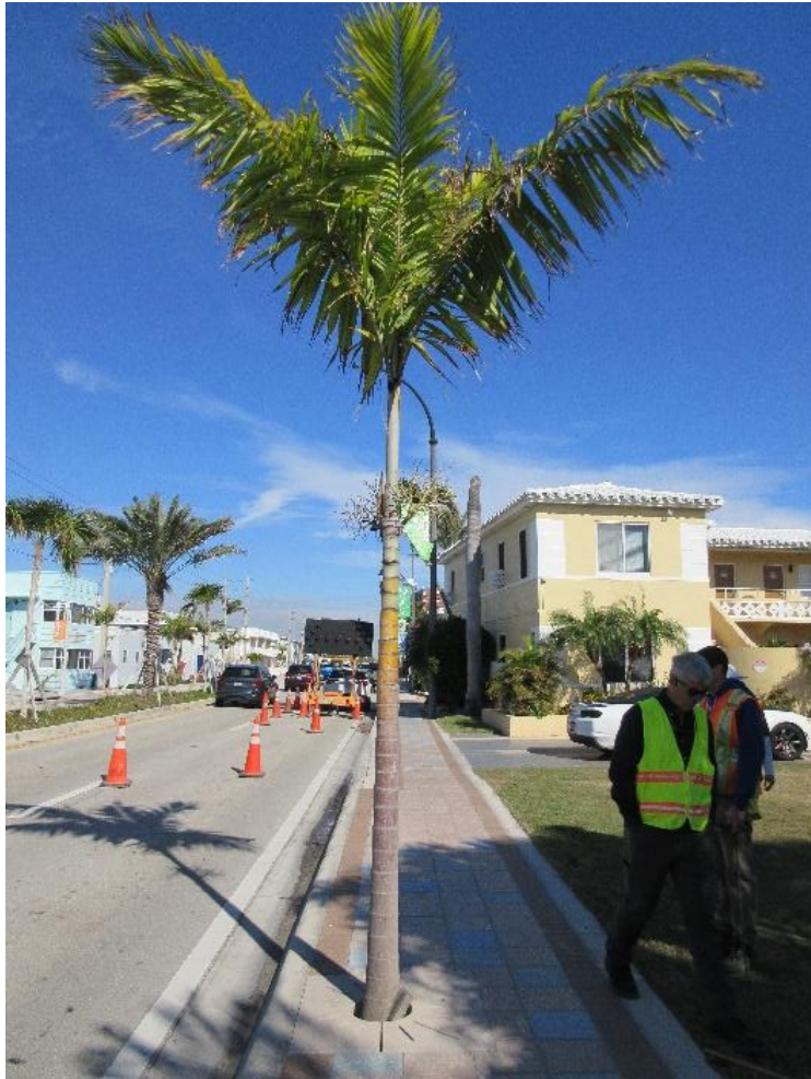
1. Back in the tree grates with stone layer
