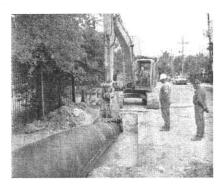
**DERM01-WASD-NLE-WEST 54" FORCE MAIN PROJECT, MIAMI-DADE WATER AND SEWER DEPT., FL.** Project included installation of approximately 9,100 LF of 54" PCCP via open cut method. Project was a design build bid thru MDWASD. The project included work within the Opalocka airport which involved extensive coordination with the air traffic tower as well as airport authorities, installation of 54" PCCP across Red Road, connection to a live 48" ductile iron force main and a subaqueous crossing.
