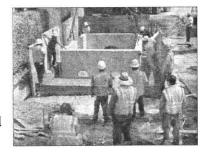
MIAMI BEACH HIGH SCHOOL "SUFFOLK CONSTRUCTION, INC." This Project consisted of relocation a live 36-inch sewer force main in 2006 for the construction of Miami Beach High School. The scope of work involved installing two (2) 36"x30" Tapping Sleeves for the installation of 2 line stops and installation of approximately 200 LF of 36" DIP with fittings.
