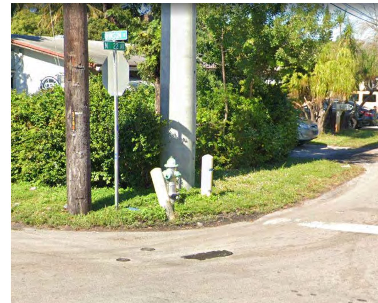
EXIST. FIRE HYDRANT 3
