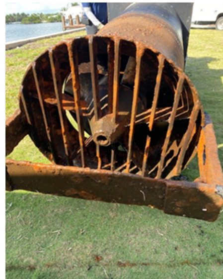
Visual Inspection of City of Hollywood Pump Station
